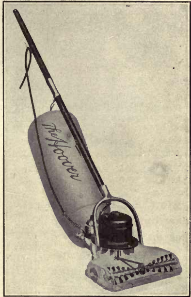
FIGURE 202.—VACUUM CLEANER DRIVEN BY AN ELECTRIC MOTOR.
